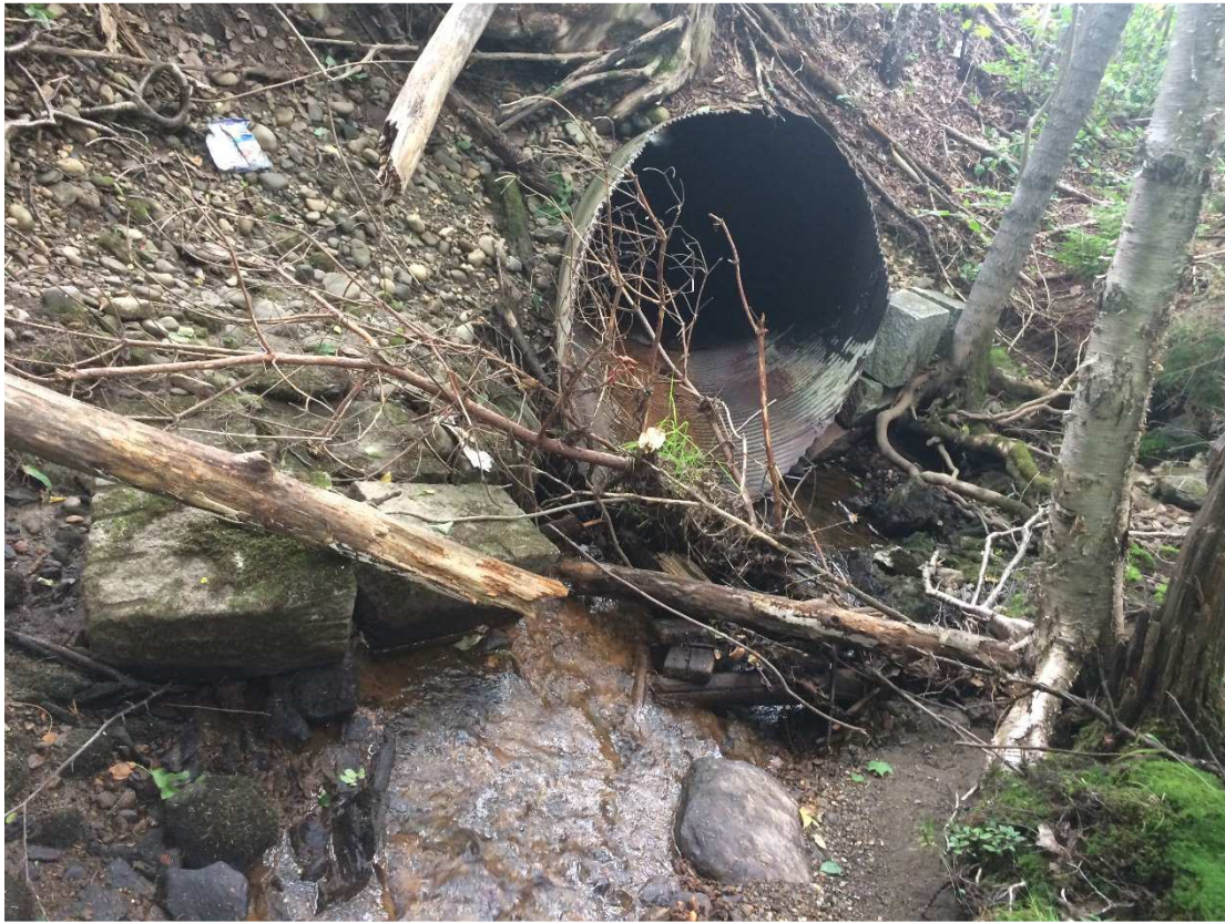
Figure 4: Inlet of Culvert
